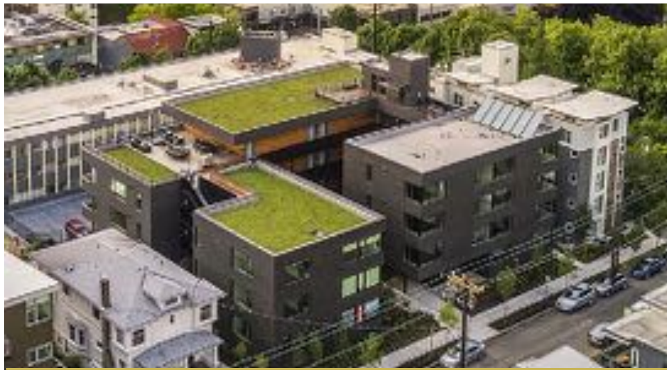
CS1 - Green Roof
