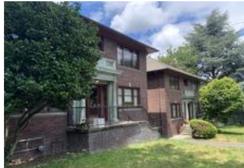
2 Raised Entry Porch
