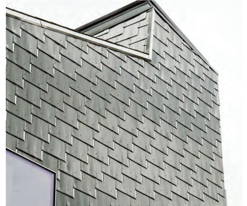
SHINGLE-LIKE SIDING PULLS FROM CEDAR SHAKE
