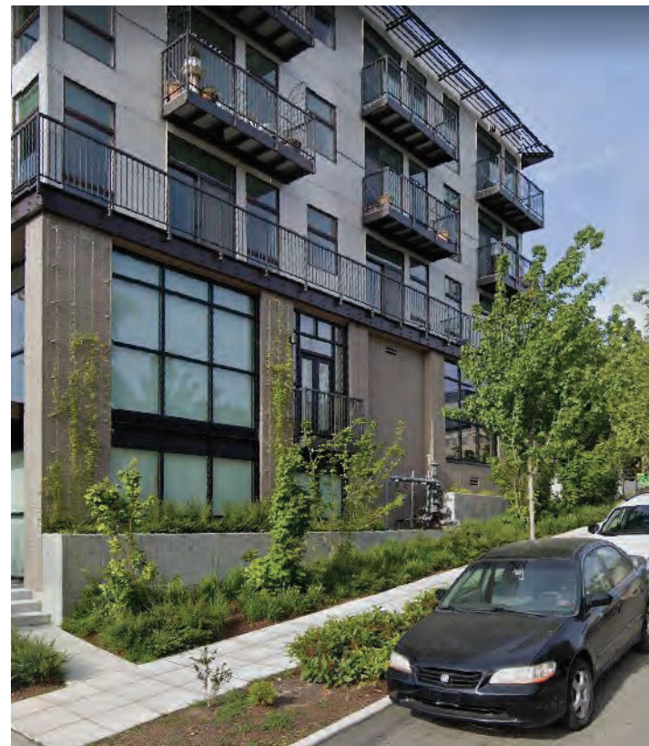
stepped landscape at building
