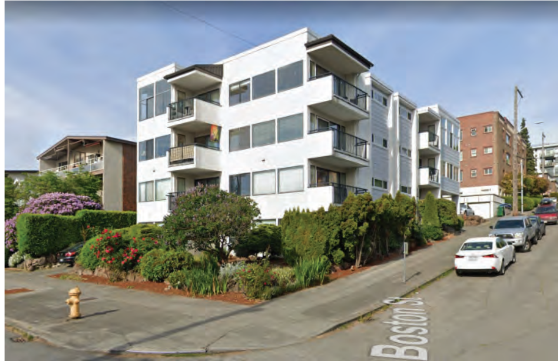
EACH UNIT HAS BALCONIES
