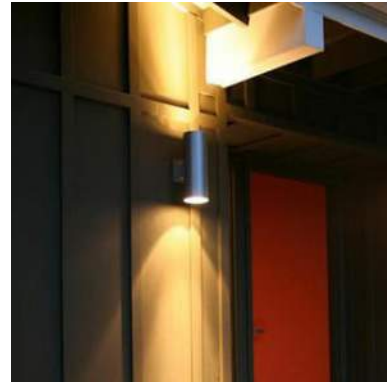
② EXTERIOR SCONCE
