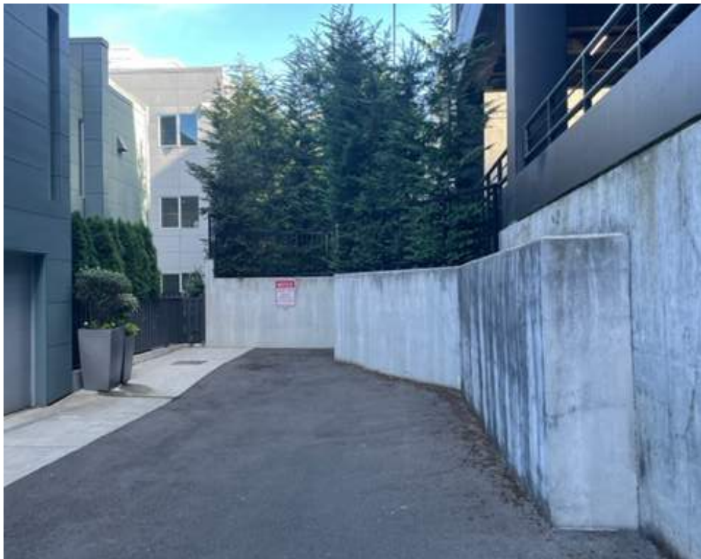
EXISTING SOUTH NEIGHBOR ALLEY CONDITION LOOKING NORTH
