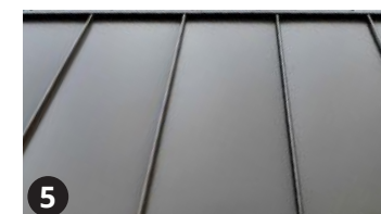
5 STANDING SEAM METAL SIDING
