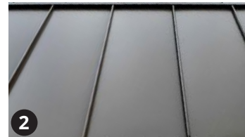
2 STANDING SEAM METAL SIDING
