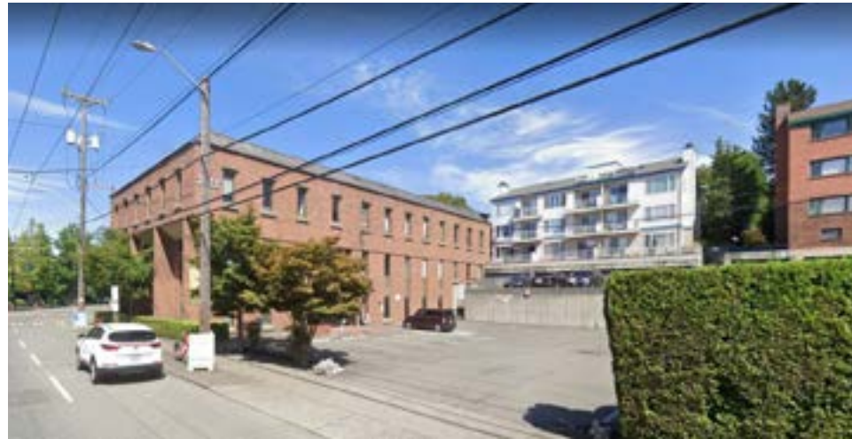
1 LOOKING NORTH ON EASTLAKE AVENUE EAST
