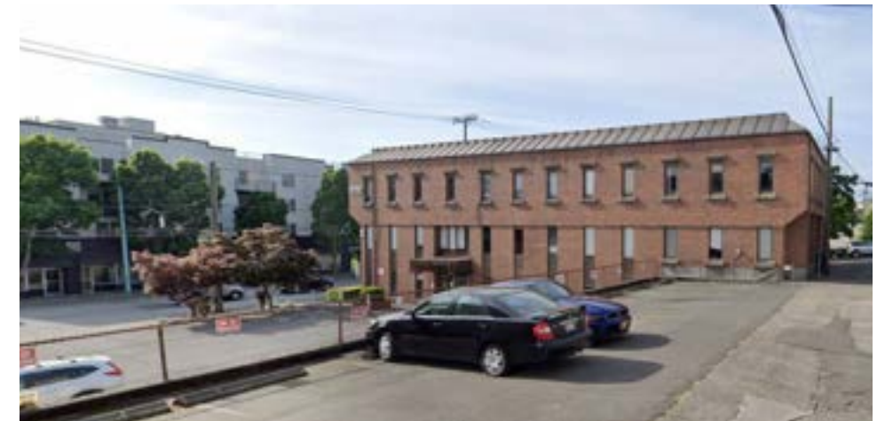
6 VIEW OF THE EXISTING BUILDING FROM THE ALLEY LOOKING NORTH-WEST
