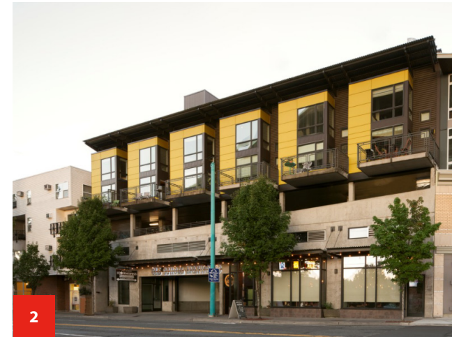
3218 EASTLAKE AVE E Concrete & Rainscreen Panel
