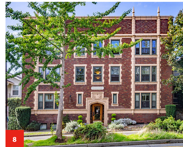
2027 EASTLAKE AVE E (HISTORIC) Brick & Stone
