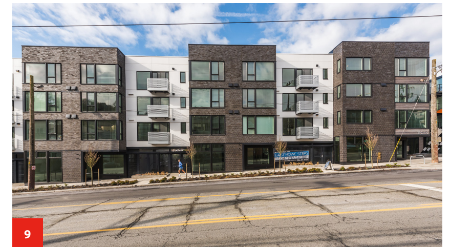
1823 EASTLAKE AVE E Brick & Fiber Cement
