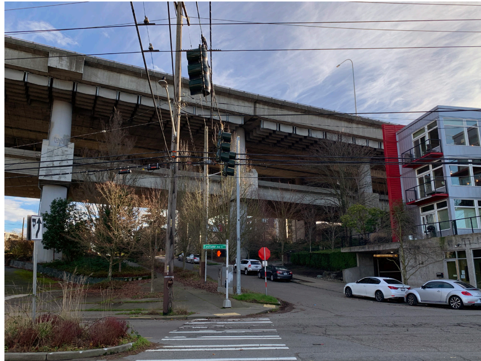
① SHIP CANAL BRIDGE
