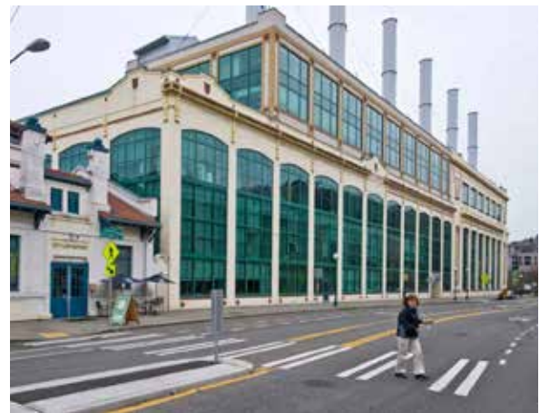
STEAM PLANT BUILDING
