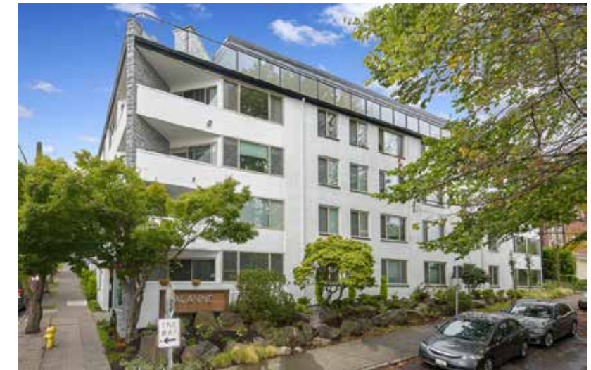
VAL ANNE | 800 Queen Anne Ave N (Renovation)
