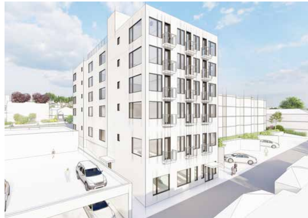
View from the Alley - Looking Southeast
