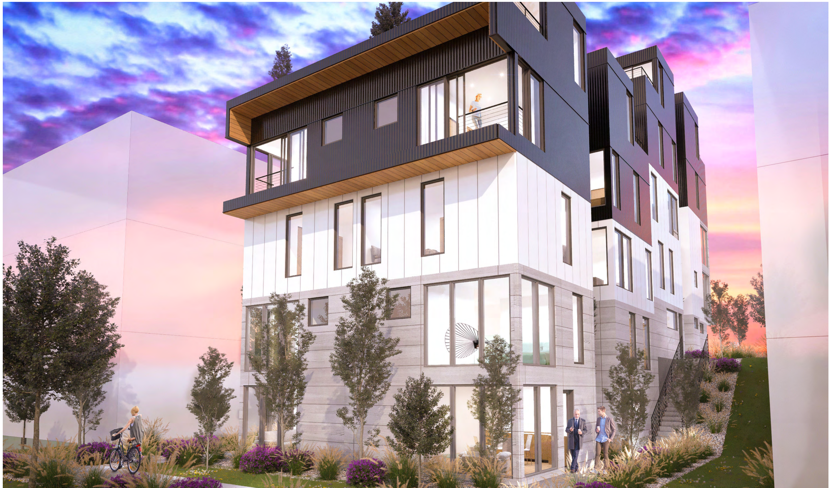
Looking NE from Street
