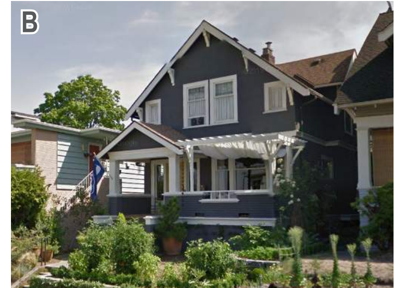
B 2352 FRANKLIN AVE E SINGLE FAMILY HOUSE PROGRAM: 1 Detached Garage
