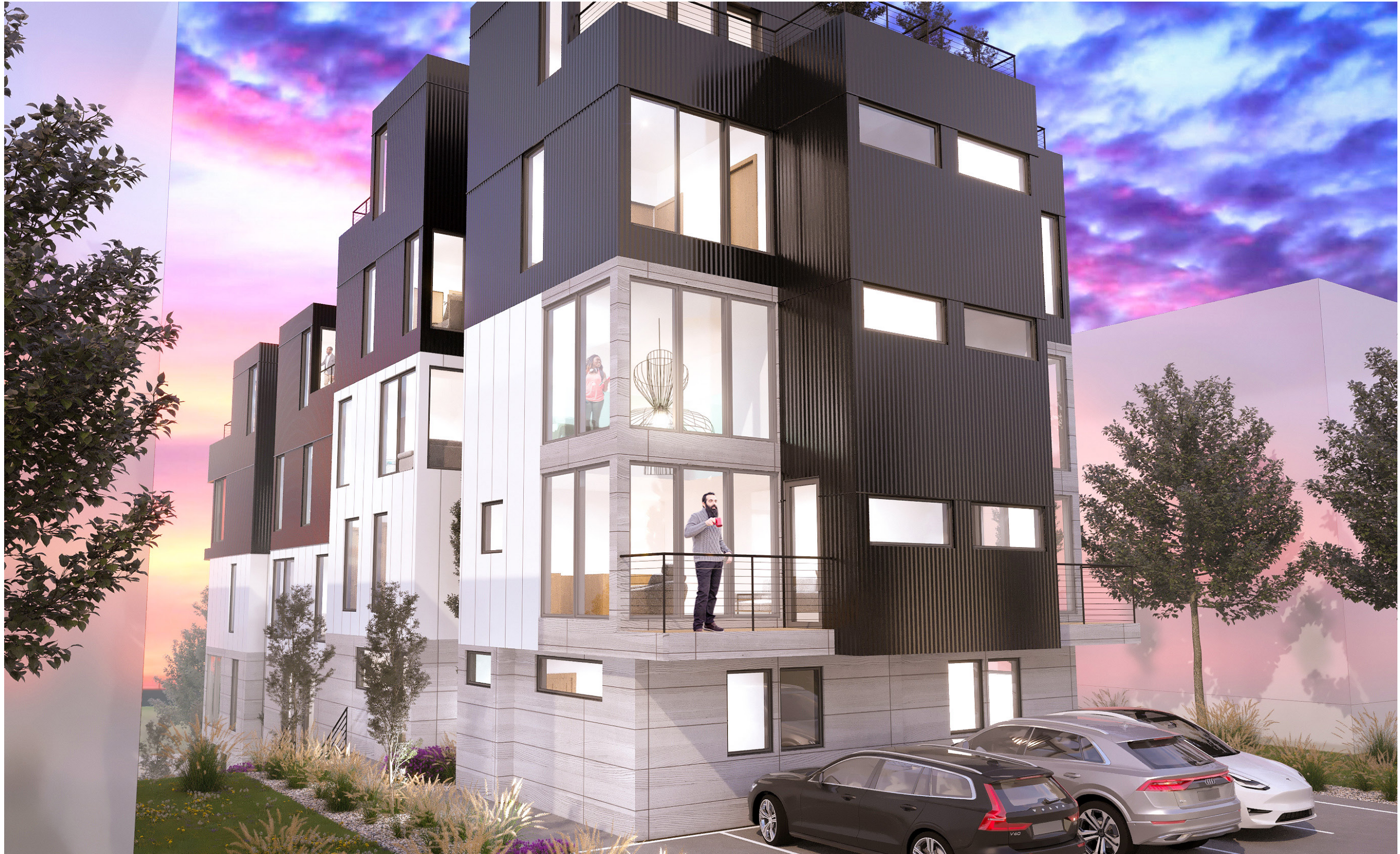
Looking NW from Alley
