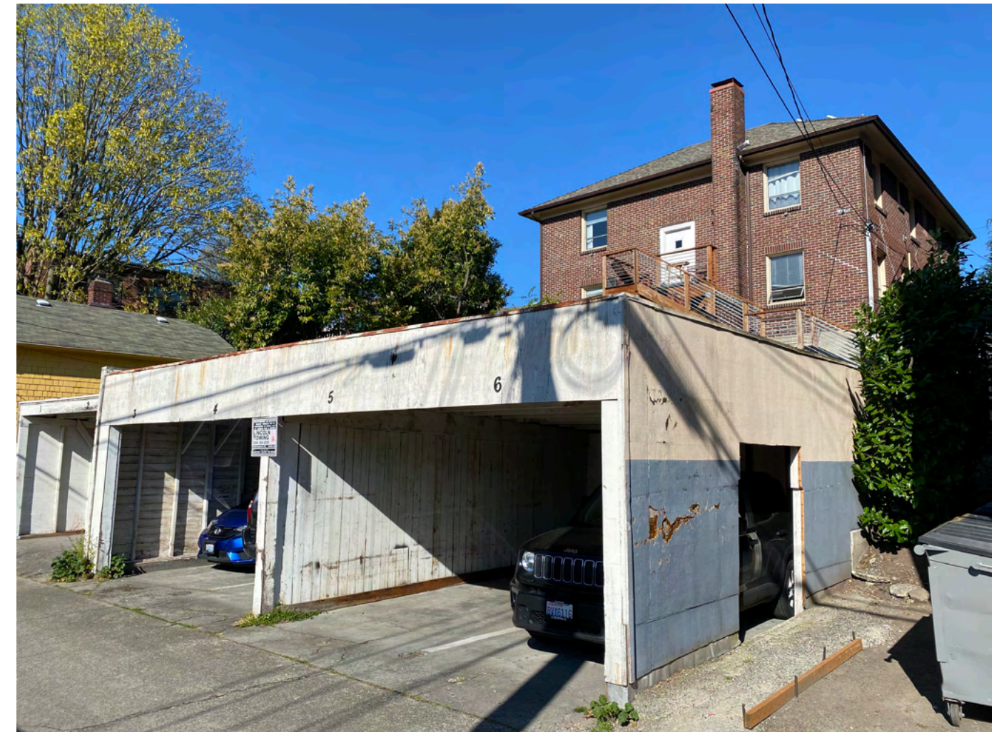
Looking NE from Alley at Existing Site. Existing Apartment to be Retained. Existing Carport to be Removed.
