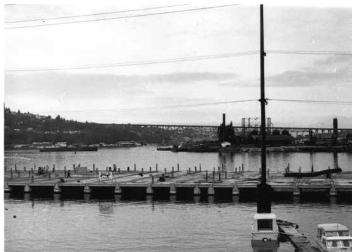
Roanoke Reef Construction. (photo credit: Seattle Municipal archives)
