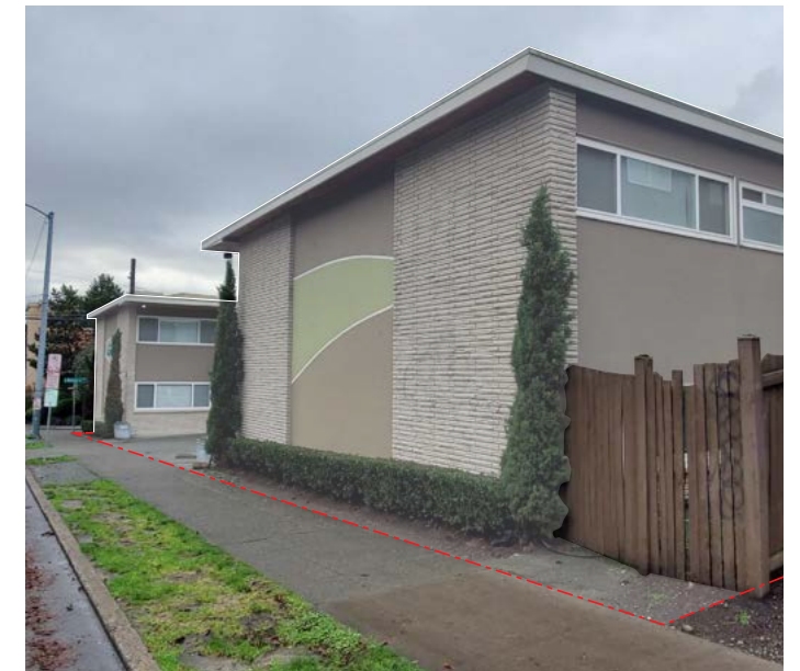
6 SIDEWALK ALONG EASTLAKE AVENUE E LOOKING SOUTH
