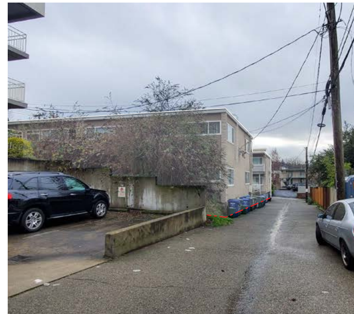
5 ADJACENT PROPERTY TO THE NORTH FROM ALLEY
