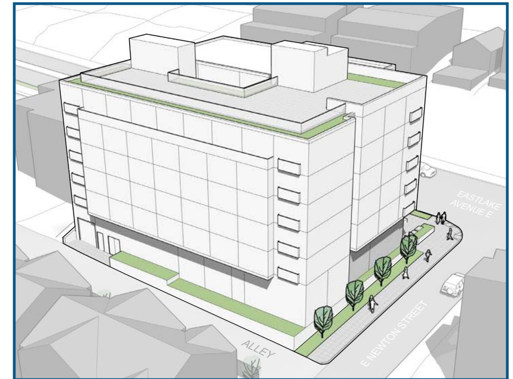
AERIAL VIEW FROM SOUTHWEST
