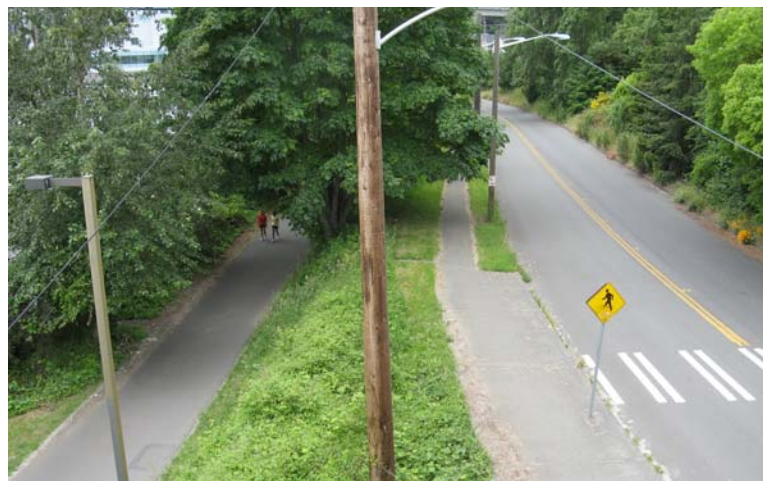
Burke Gilman Trail and NE 40th from University Bridge.
