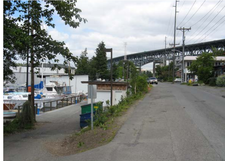
Fairview Avenue East north of Fairview Park.
