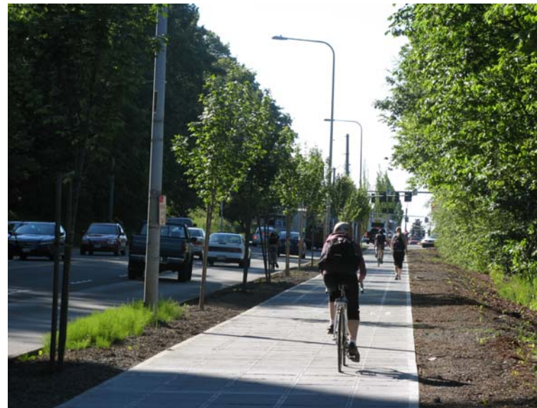
New sidewalk along Westlake Avenue North.
