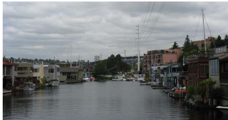
Fairview Avenue East right-of-way from the Roanoke Street End.
