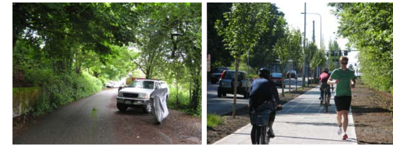
LEFT: Shoreline right-of-way extending from under Fremont Bridge south to end of new sidewalk on Westlake. RIGHT: New sidewalk on Westlake Avenue, south of Fremont Bridge.
