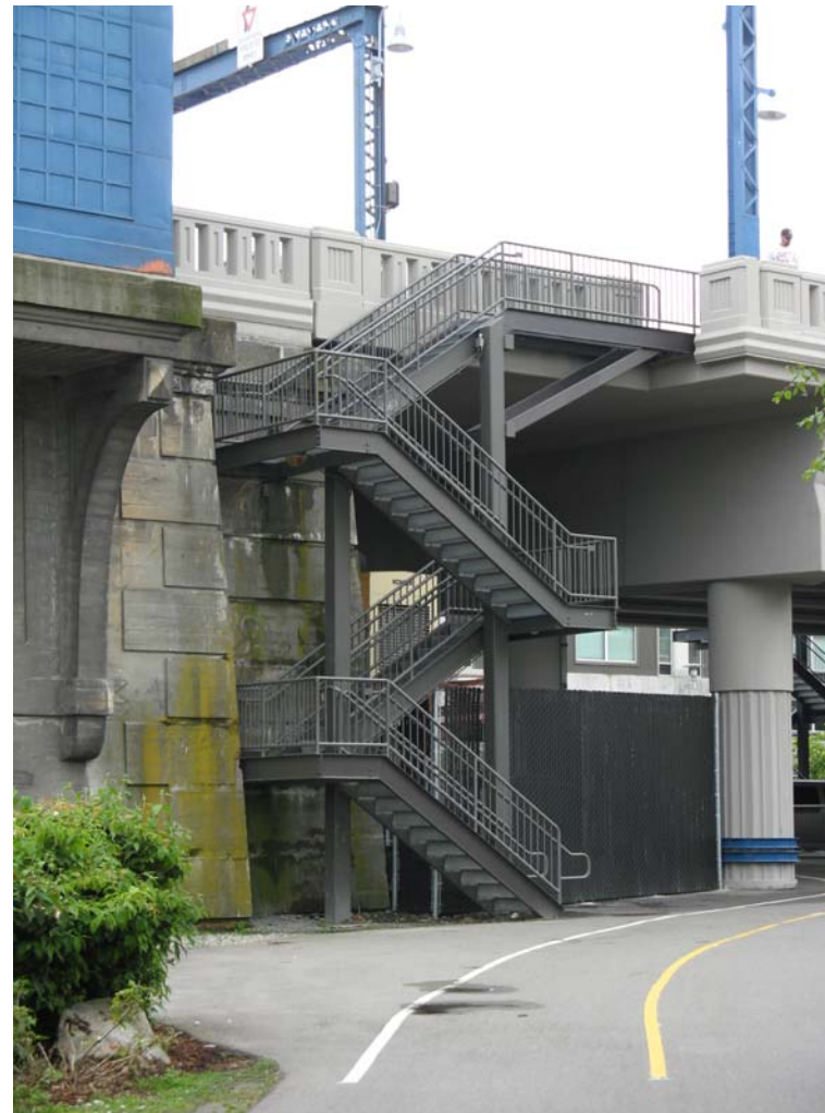
Existing stairway from shoreline pathway to bridge deck.
