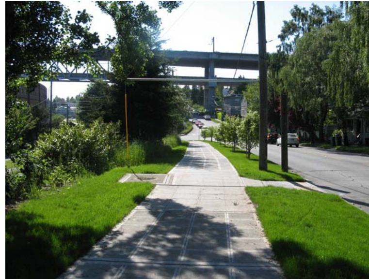
New sidewalk at Peace Park/NE 40th Street.
