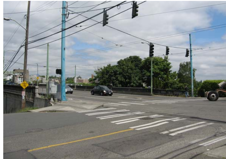
South end of University Bridge from Fuhrman Avenue East.
