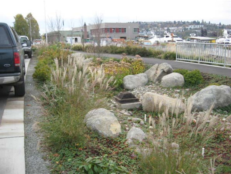
Drainage basin cleansing on Fairview Avenue East, near Ward's Cove.
